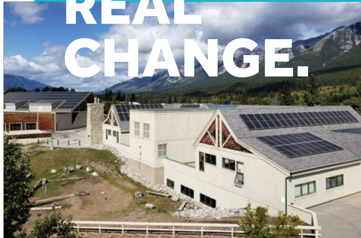
Solar PV array at Canmore Collegiate High School.
