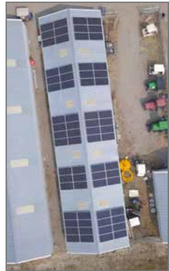
Golf Course Maintenance Building
