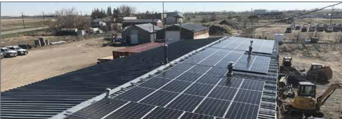
Raymond Public Works Shop
