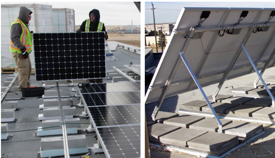
Figure 18: Ballasted solar PV racking on flat roofs
