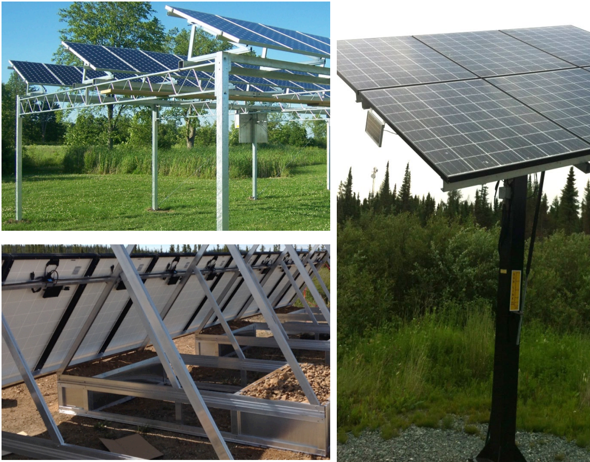
Figure 19: Top-of pole and frames used for ground-mounting solar PV systems Photo: Green Sun Rising (top-left, bottom-left); Dave Lovekin (right)
