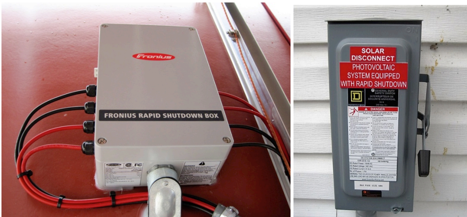
Figure 11: Rapid shutdown device (left) and DC disconnect with appropriate labeling (right) Photo: SkyFire Energy and Green Sun Rising
