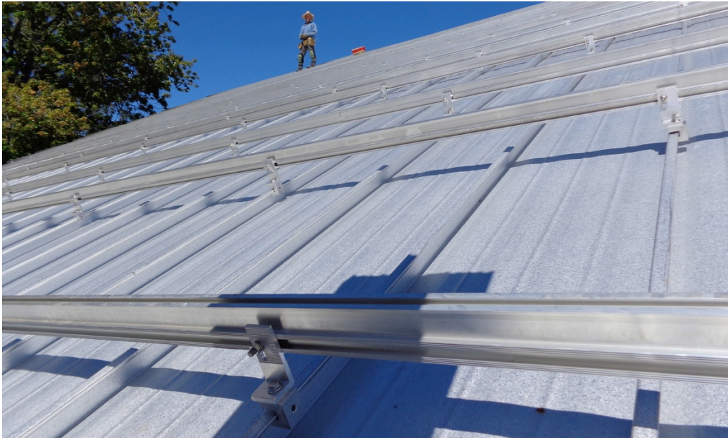
Figure 17: Solar PV racking on lightweight metal roof
