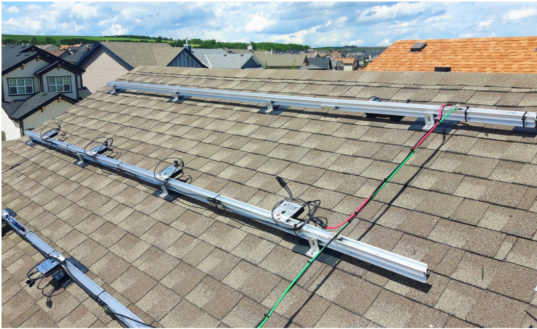
Figure 16: Solar PV racking on sloped asphalt roof
