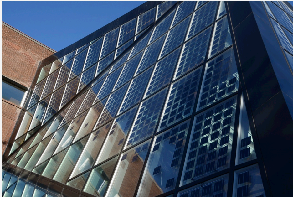
Figure 25: Building-integrated photovoltaic system
