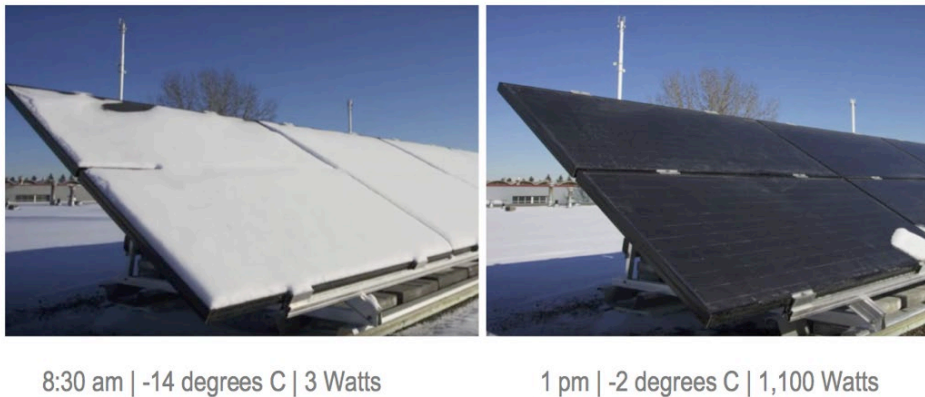
Figure 15: Snow accumulation on solar PV modules
