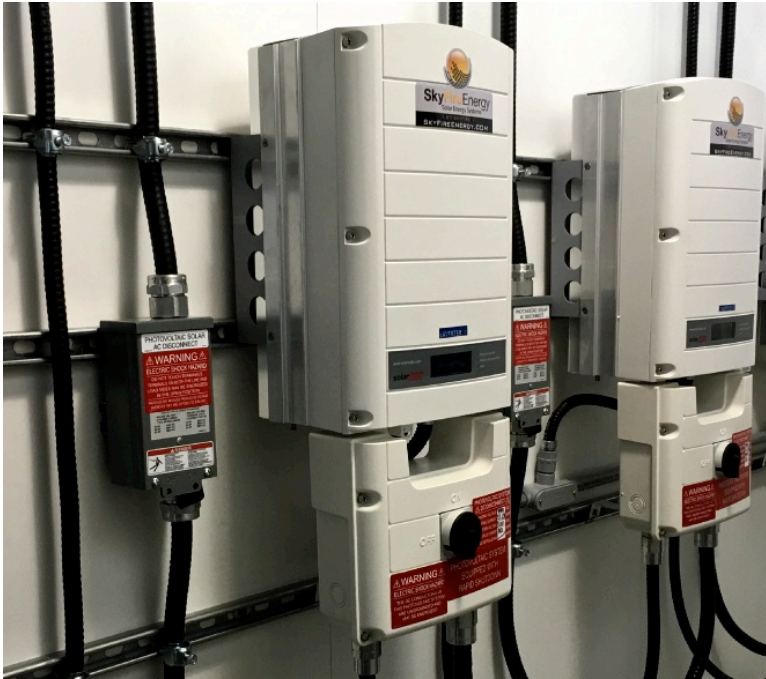
Figure 10: Solar PV system disconnects and electrical panels Photo: SkyFire Energy
