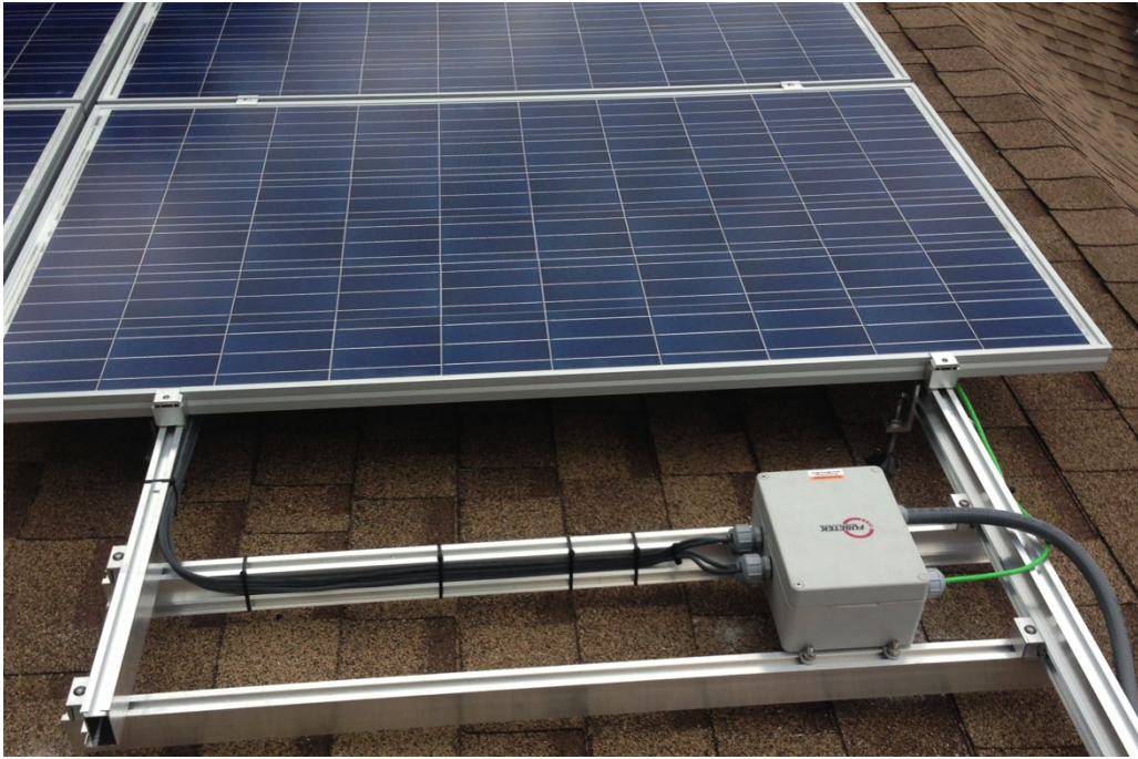
Figure 9: Solar PV system cabling and combiner box
